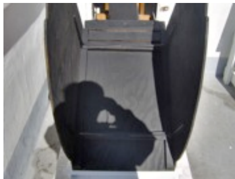
Inside of new hatch for Stuhlinger.
